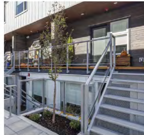
179.1 Handrail and Guardrail
