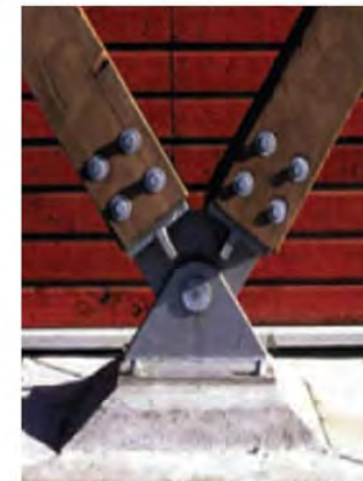
174.3 Timber with Metal Fastening
