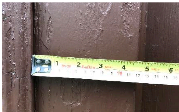
Original trim dimension - close to 6" with backband, and 4.5" without)
