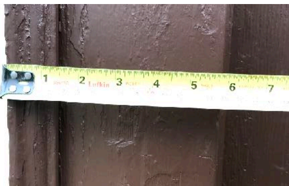
Original trim dimension - close to 6" with backband, and 4.5" without)
